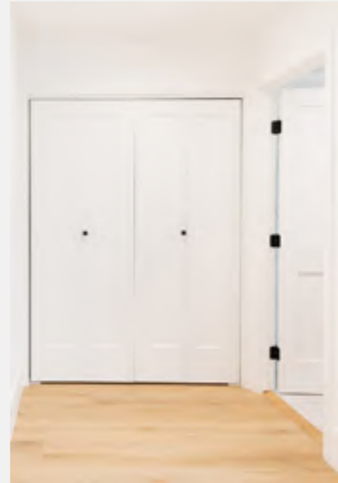
High hollow core Hume flush panel with painted finish to linens (match internal doors).
